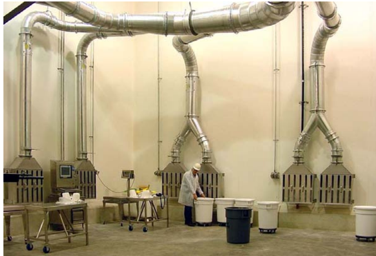
Figure 5, Typical Hood System
